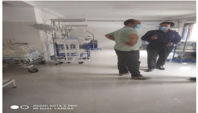
Under Construction SNCU at CHC Uri
