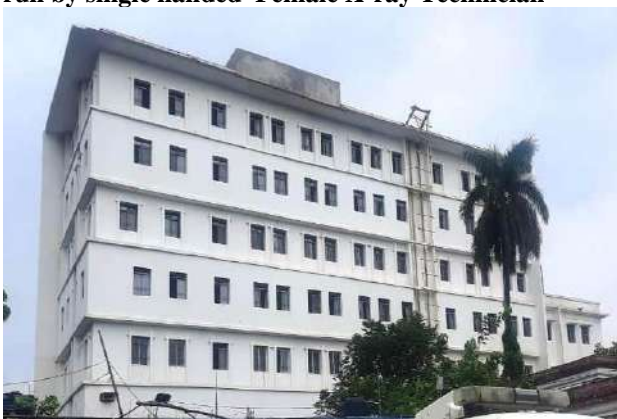
New Building under Construction for DH Vaishali
