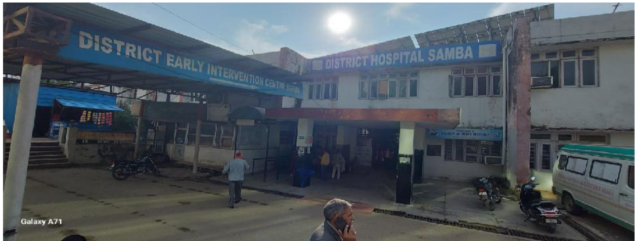
The District Hospital Building Samba is not in a good condition
