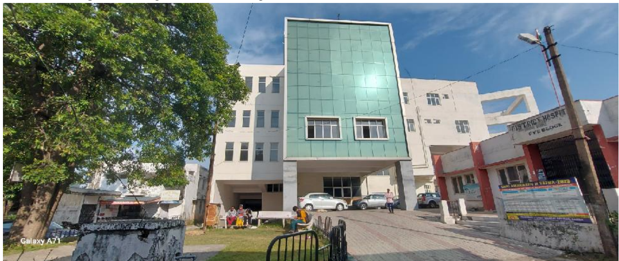
Newly constructed building for DH Samba but has not been handed over because of construction faults
