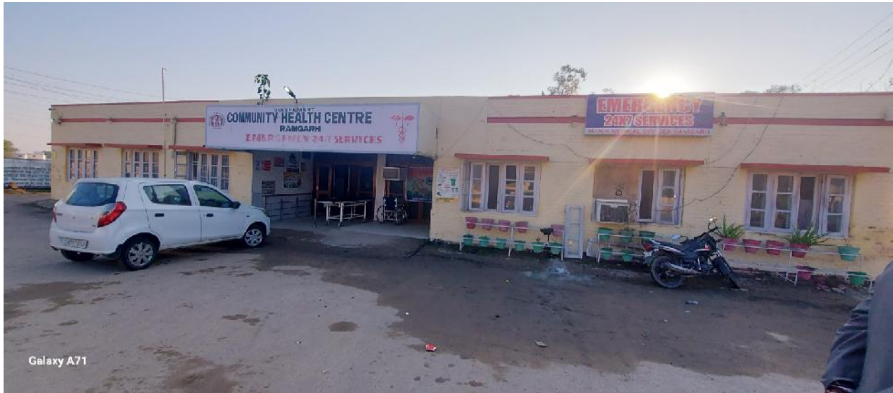
Well maintained building of CHC Ramgarh
