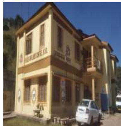
New building PHC-HWC Kud
