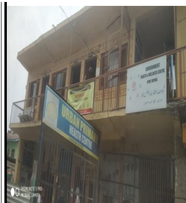
UPHC Sopore in Rented Building
