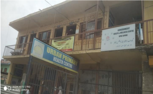
UPHC Sopore in Rented Building with Limited
