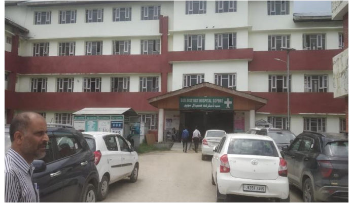
SDH Sopore Building
