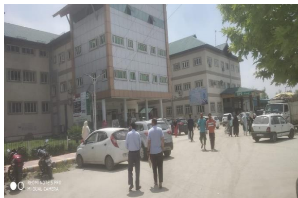
New DH Building at Ganderbal
