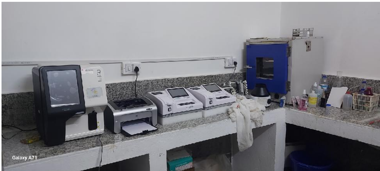
All the newly Analyzers installed at CHC Atholi are non-operational due to some technical errors
