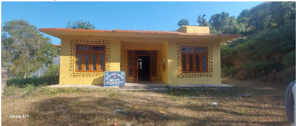
SC Maslote is located far flung area near a Jungle and is without a boundary wall
