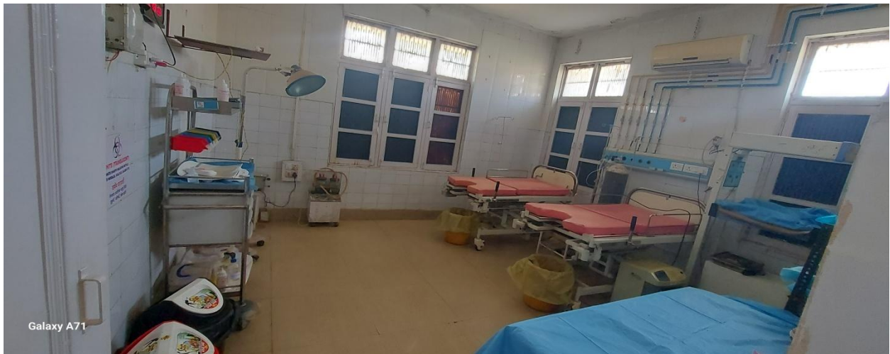
The condition of labour room at CHC Hiranagar is not good due to the space constraint and as such no attached washroom.
