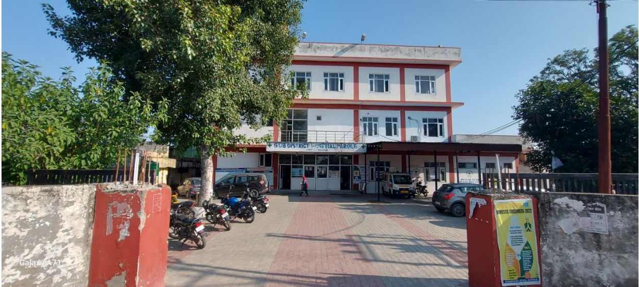
Well maintained building of CHC Parole of district Kathua
